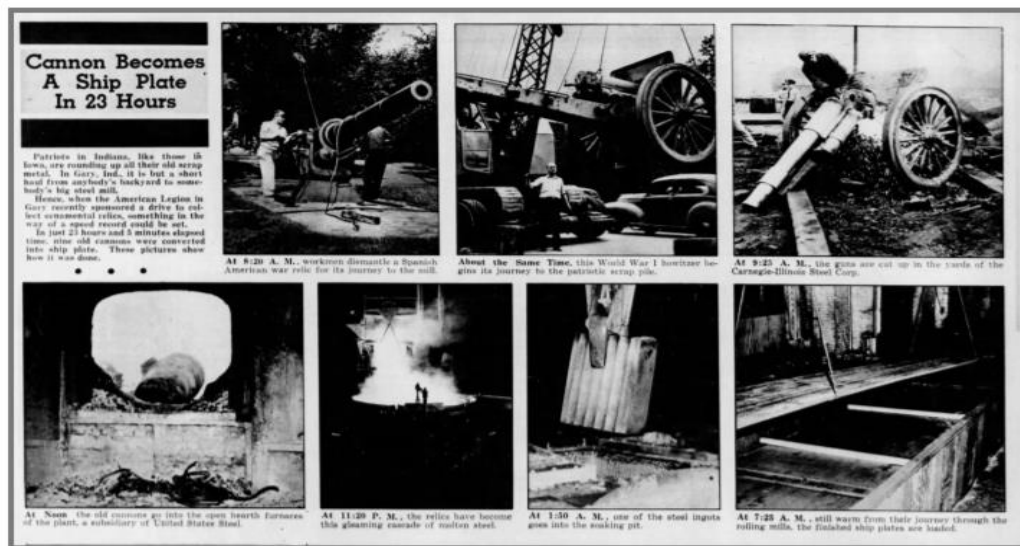
Figure 10. A feature in the October 11, 1942, edition of The Des Moines Register depicts the transformation of a World War I cannon into a steel panel for installation on a new ship.
